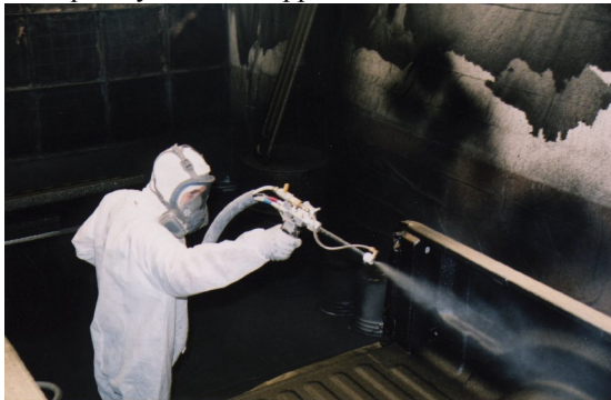
Gatorhde low-pressure polyurea hybrid applied onto a truck
