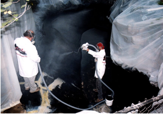
Gatohyde LP (RF85) applied as a pond liner at the Tulsa Zoo
