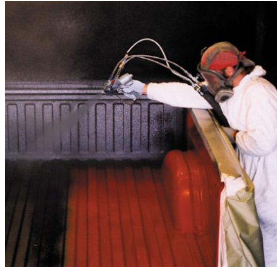
A spray-in bedliner is applied using high-pressure equipment and material
